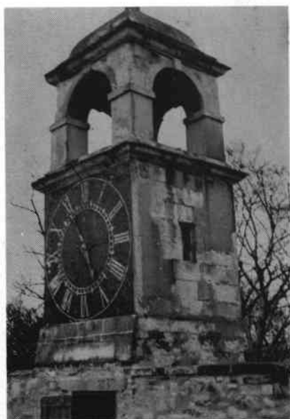
Turret clock at Gilling Castle which I have been repairing.
