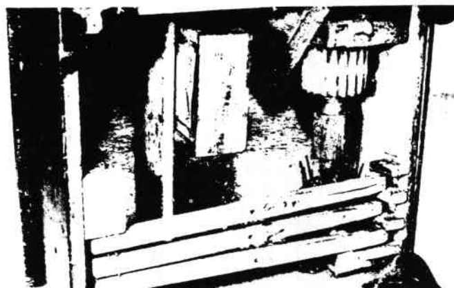
Figure 2. The mechanism of "The Dandy Fiddler". This is not at all typical and suggests Black Forest origins. The tune card is only readable when the mechanism is dismantled!
