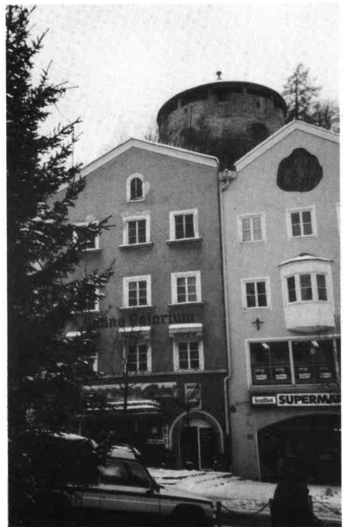
The Burghertower above the rooftops, housing the organ. Note the opening for the sound to speak out. The organ is linked electrically to the console at street level, to the left of these shops.
