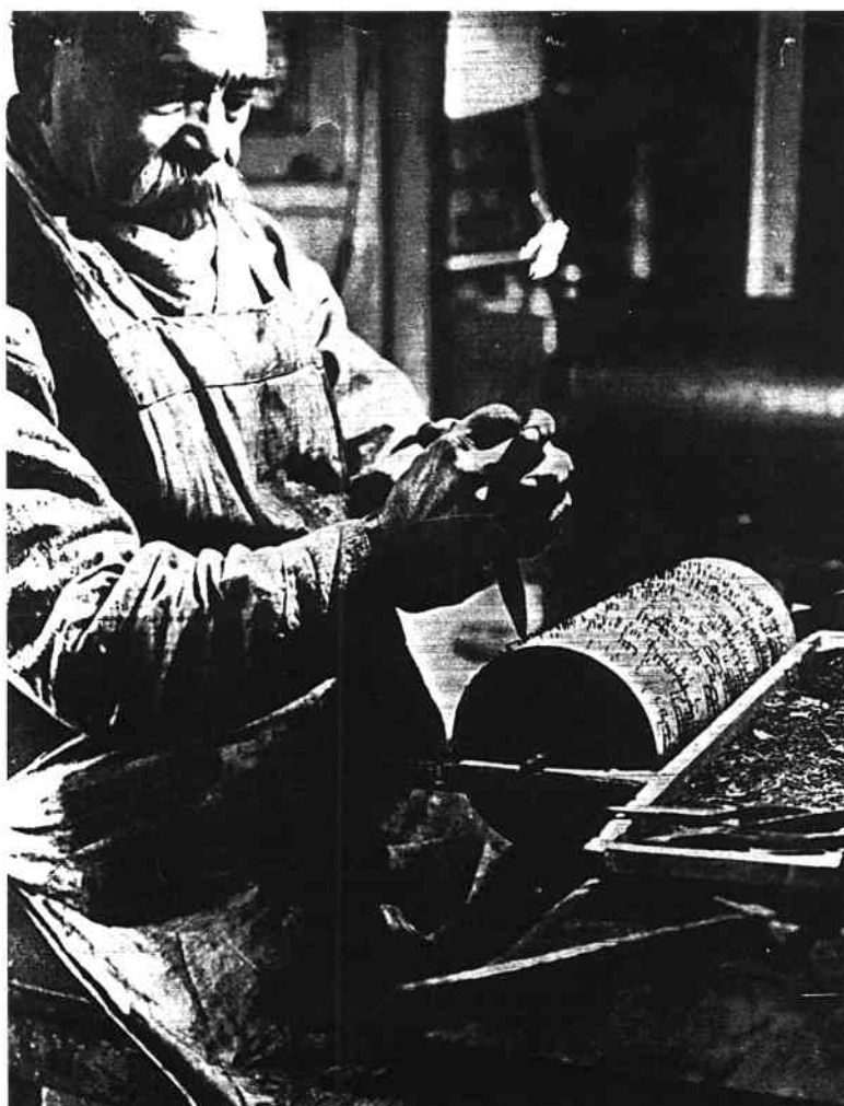
Fig.5. Photograph of Luigi V. Tomasso pinning a barrel in his workshop.
