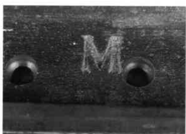
Fig. 5. Foundry mark M cast in both comb bases.
