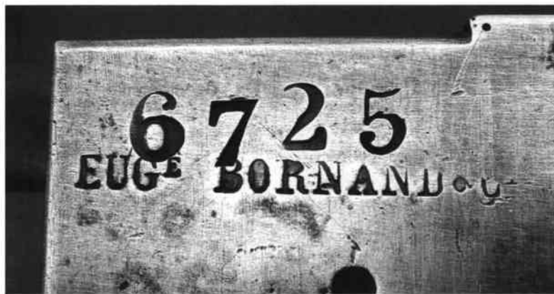
Fig. 8. The one-piece stamp of EUG E BORNAND & CIE (heavy at bottom left and weak at top right so " & C" is almost lost). Langdorff's 6725 stamp is badly aligned and also weak at the top, - and applied with scant care about the Bornand. This 8" cylinder 4-air box has all the Langdorff characteristics, including, scribed on the bass end cylinder cap, the serial number 6725 and the gamme number and year, 444/52. The year had to be stated because their gamme numbers reverted to 1 nearly every year, presumably to avoid exceeding three digits.
