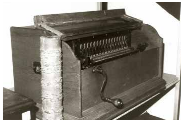
Fig 6: The 32 note Grand Roller Organ. Case measures overall, 24 \frac{3}{4} " x 15 \frac{3}{4} " X 13 \frac{1}{2} " high. Roller measures 13 \frac{1}{8} " by 2 \frac{1}{2} "
