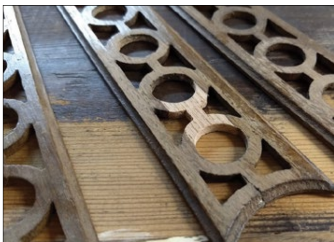
A round rosette shape had to be replaced on one of the columns so a new one was carved and fitted onto the column.
