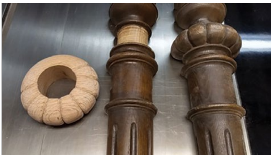
A round rosette shape had to be replaced on one of the columns so a new one was carved and fitted onto the column.
