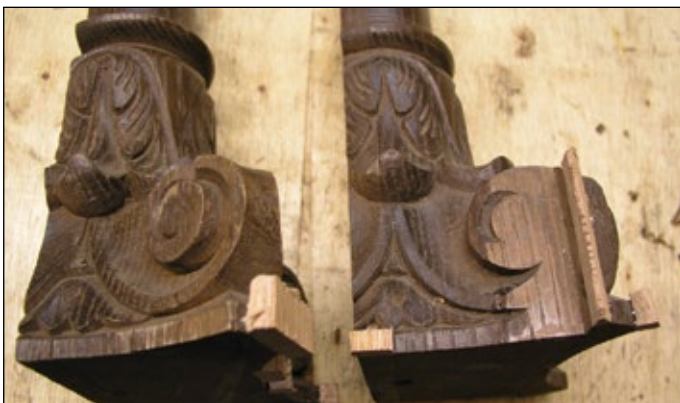
The door corbels are shown in the process of patching new wood into places where it was missing or chipped.
