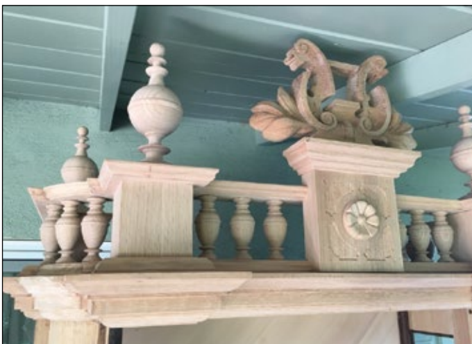
A photo showing finished turned spools and finials in what will be their final positions.
