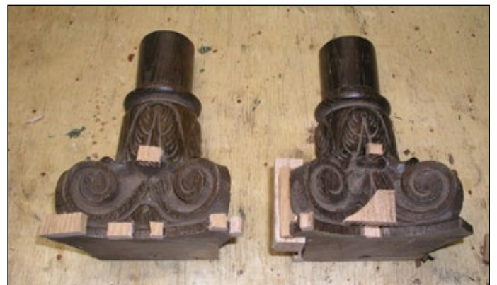
The door corbels are shown in the process of patching new wood into places where it was missing or chipped.
