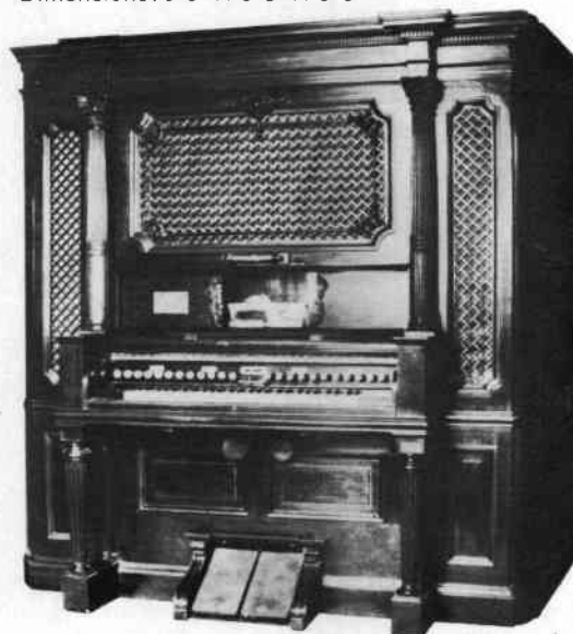
Model F No. 5952 with custom made oak case to match Tudor Minstrels gallery of Sussex stately home for which it was destined in 1912. Retubed and pneumatically restored 1976/77, this instrument is unique. Plays on 58 and 116 note rolls. Dimensions: 7' 6" x 6' 6" x 3' 3"
